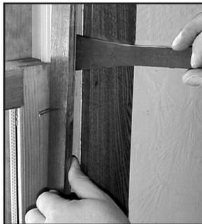
**Note:** In some applications, removal of the stop may not be necessary. Depending on the age of the window, you may have to remove metal or vinyl jambliners.
