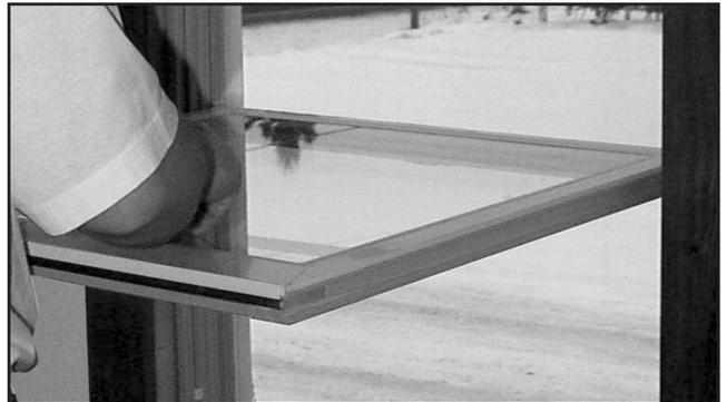
11. Tilt the sash upward until the tilt latches engage in the jambliner. Allow sash to drop and engage clutch mechanism. Repeat procedures 7 through 9 to install lower sash (using inside track). Both sash should fit snug against the jambliner.
