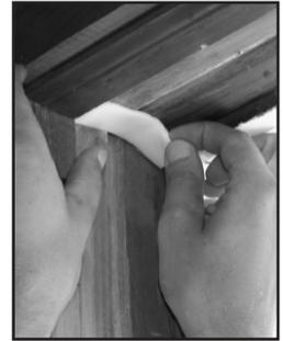
5. The metal clips are to be positioned against the jamb, approximately 4" down from the head jamb and 4" up from the sill. Attach these clips into place using the supplied #7 x 7/8" screws. Clips should be installed level and tight to inside stop.
